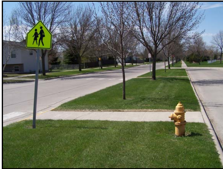
Figure 18. Sidewalks without curb ramps within the turnout lane boulevard.
