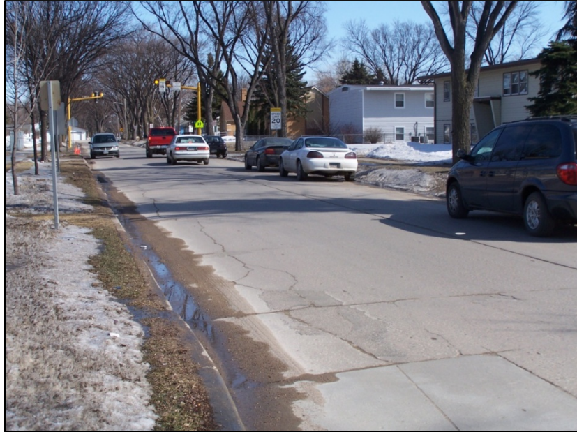
Figure 4.3. Parking on 13 th Ave. S. during dismissal
