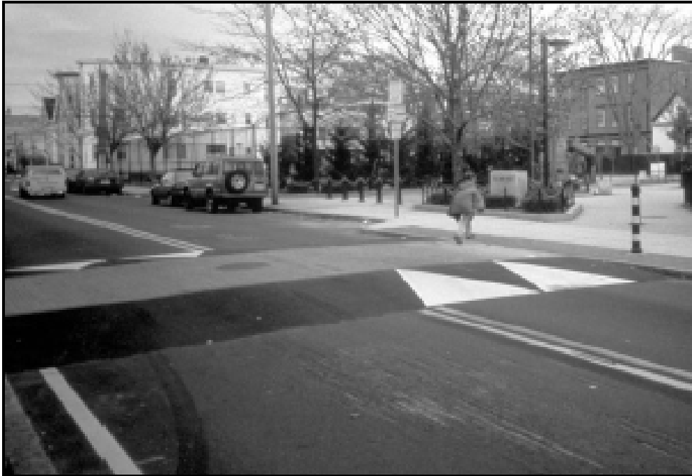
Figure 17. Example of raised crosswalk
